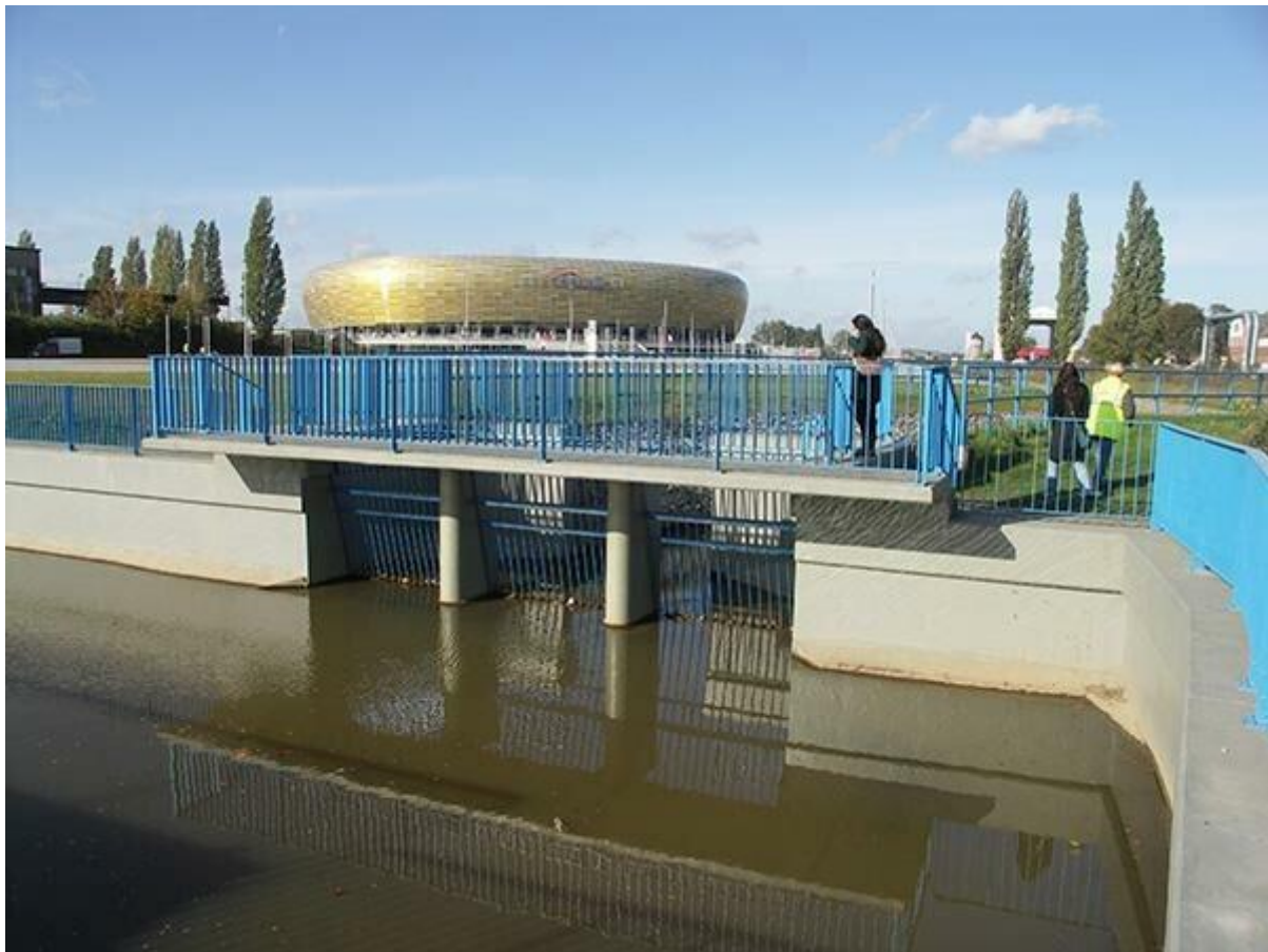
Figure 25: A Drainage of the area for the stadium as part of the Gdańsk Bay Water Protection - construction and modernization of the rainwater drainage system in Gdańsk. Photo by the City of Gdansk
