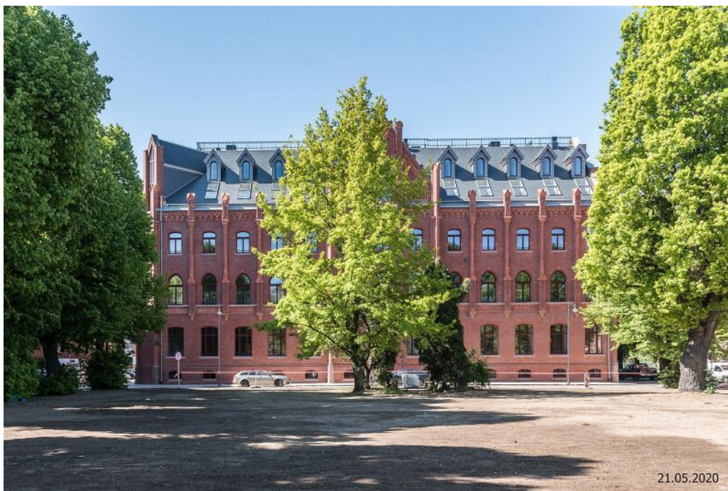
Figure 27: View of the revitalized former City Gymnasium in Gdańsk at ul. Lastadia 2 modernized 'neighbor'. Photo by Gdańsk Waters
