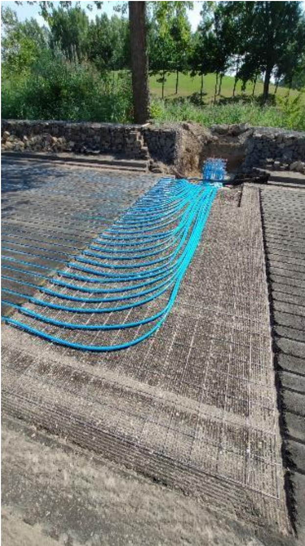
Figure 13: Tubes coming together in the so-called collector put
