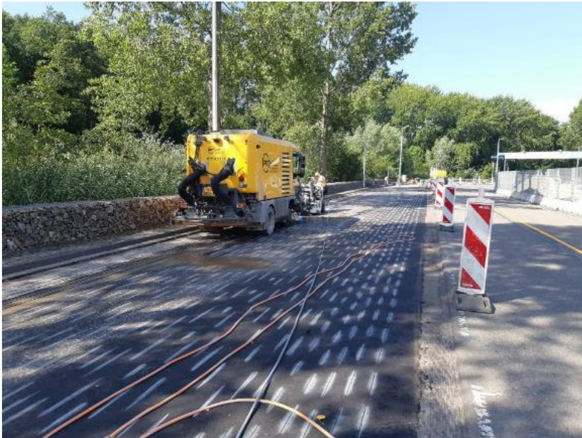
Figure 11: Milling and cleaning the pavement
