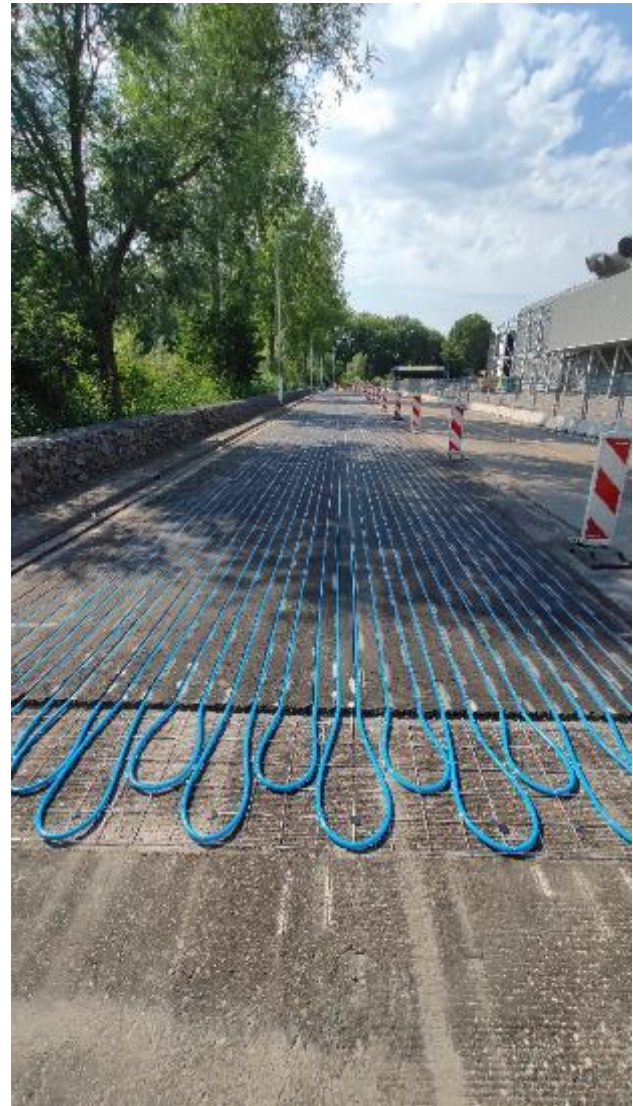
Figure 14: Overview of the tubes with the loops
