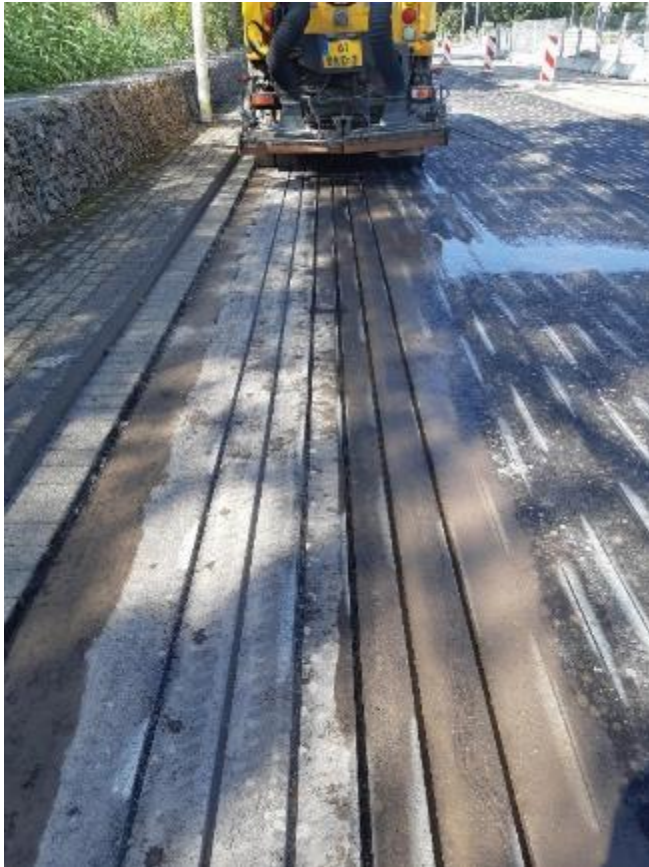
Figure 9: Milling the pavement
