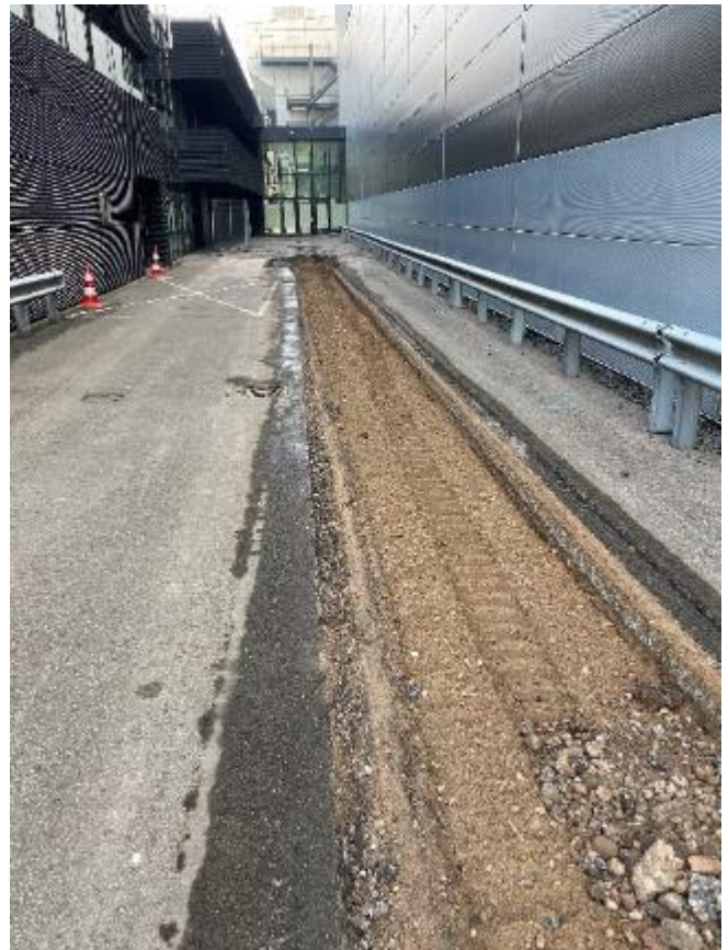
Figure 10: Digging the ground for the main piping to Ahoy
