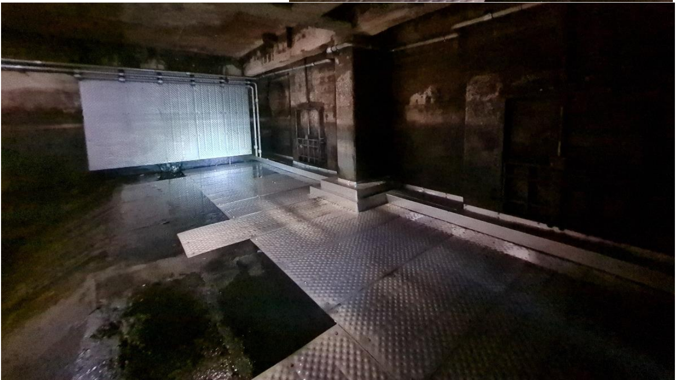
Figure 14: Heat collecting panels inside the pumping station on the floor and the wall of the basin
