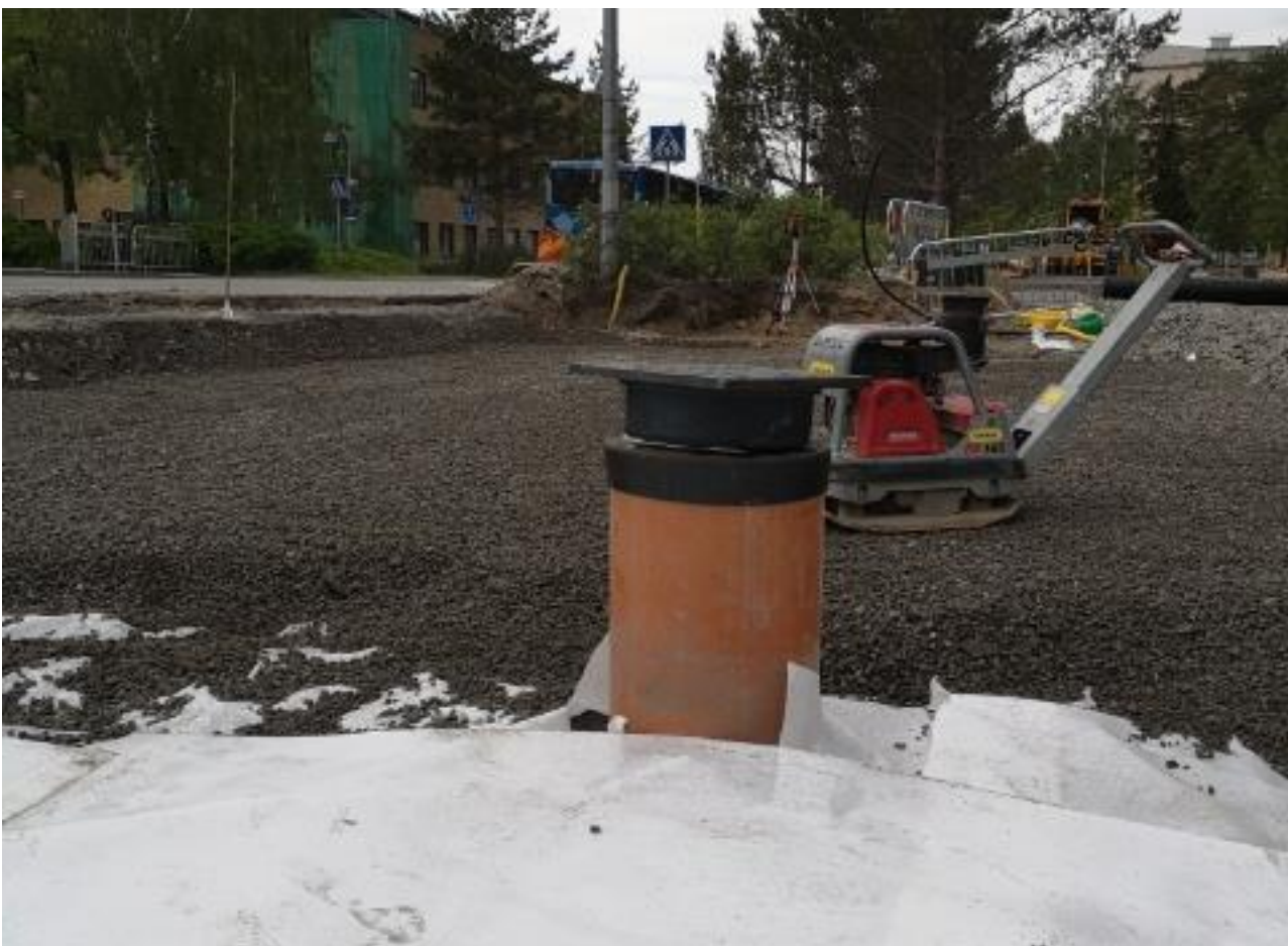
Picture 9. Non-woven cloth and drainage bed
