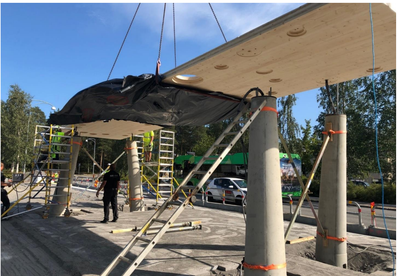
Picture 15. The first plate is mounted
