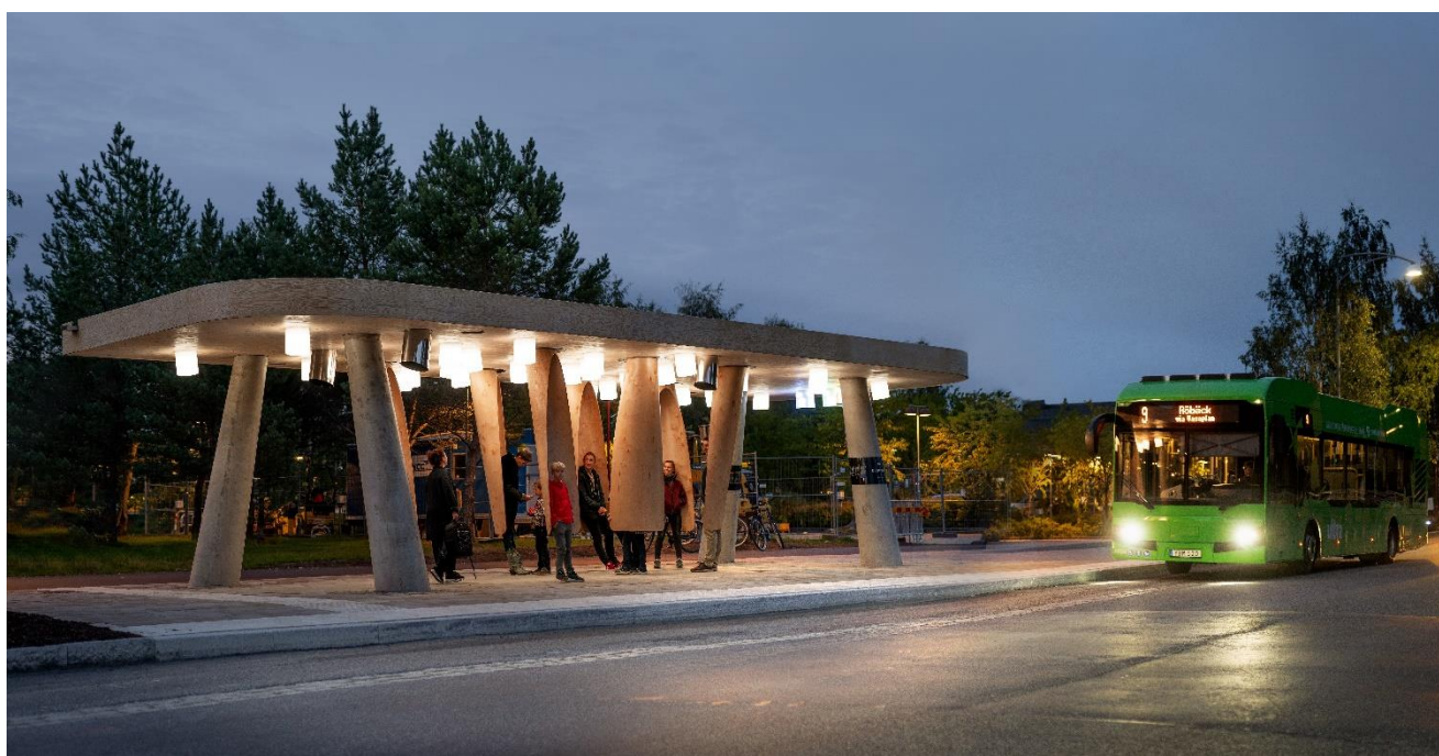
Picture 5. The smart bus station senses when a bus is on approach
