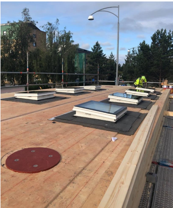
Picture 19. Light inlet mounted
