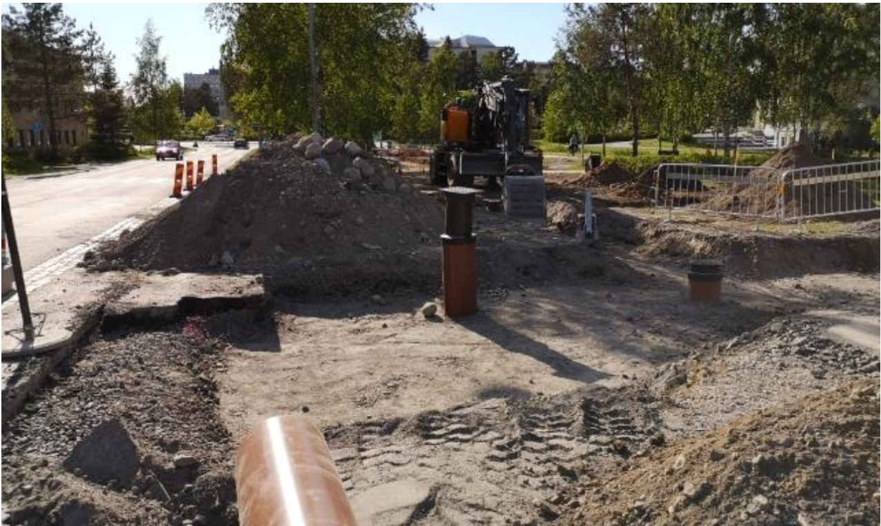
Picture 8. Drains with supervisory well are built
