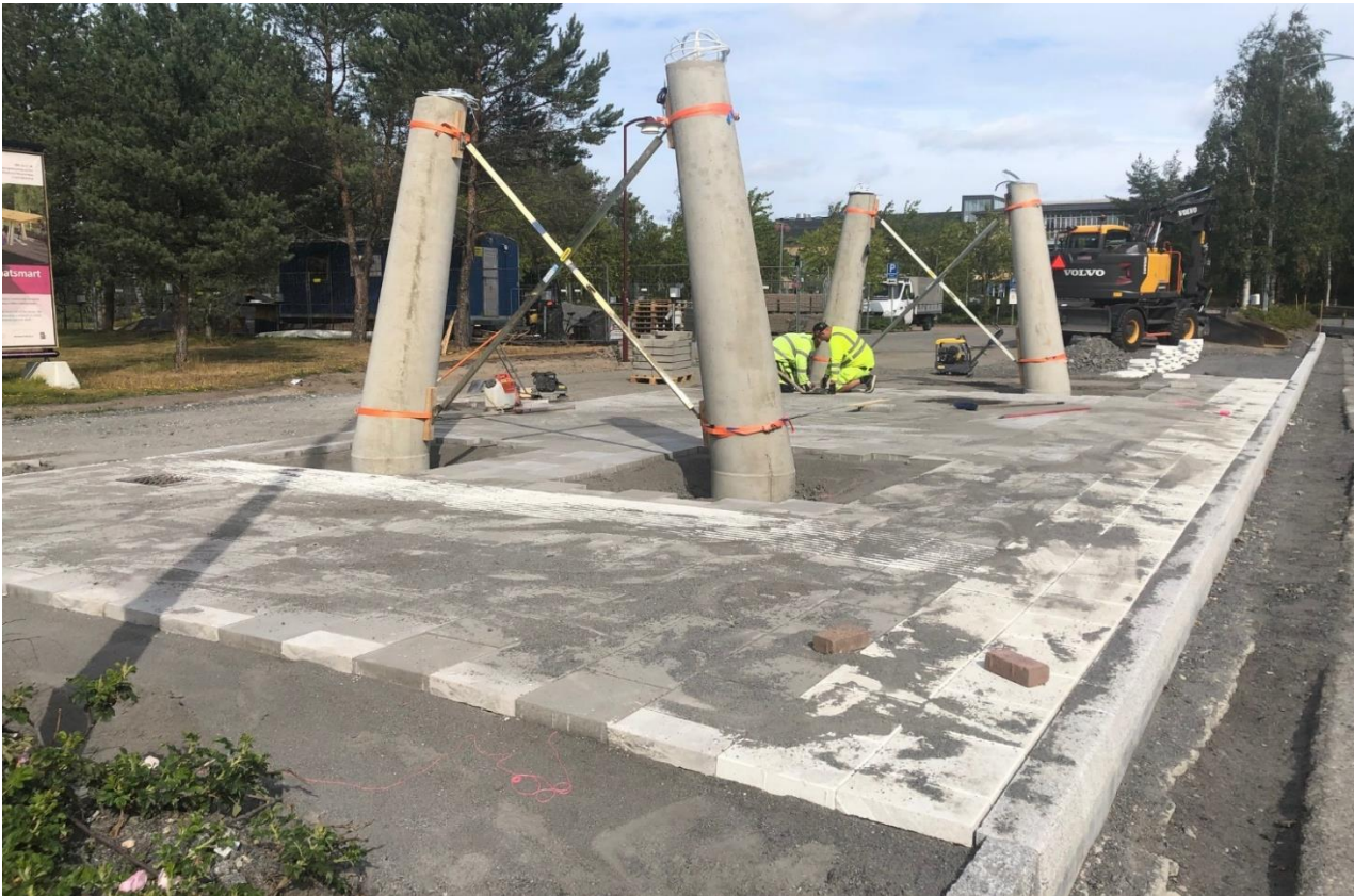
Picture 14. Tiling complete and wiring in pillars
