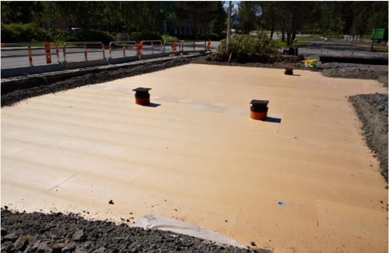
Picture 10. Insulation of surface
