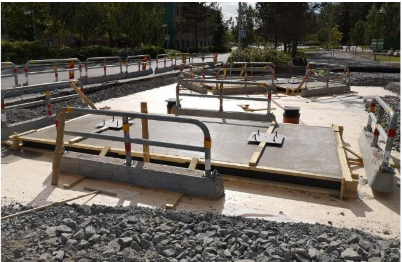
Picture 11. Casting of pillar foundations
