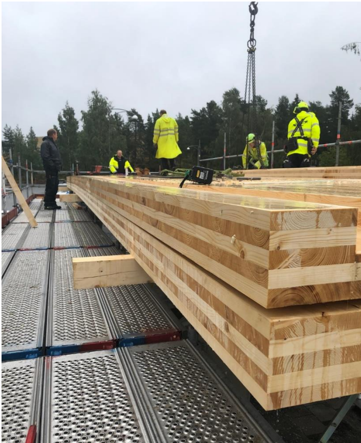
Picture 18. Fitting of plates
