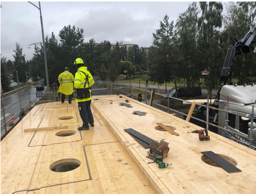
Picture 17. The second top plate is mounted
