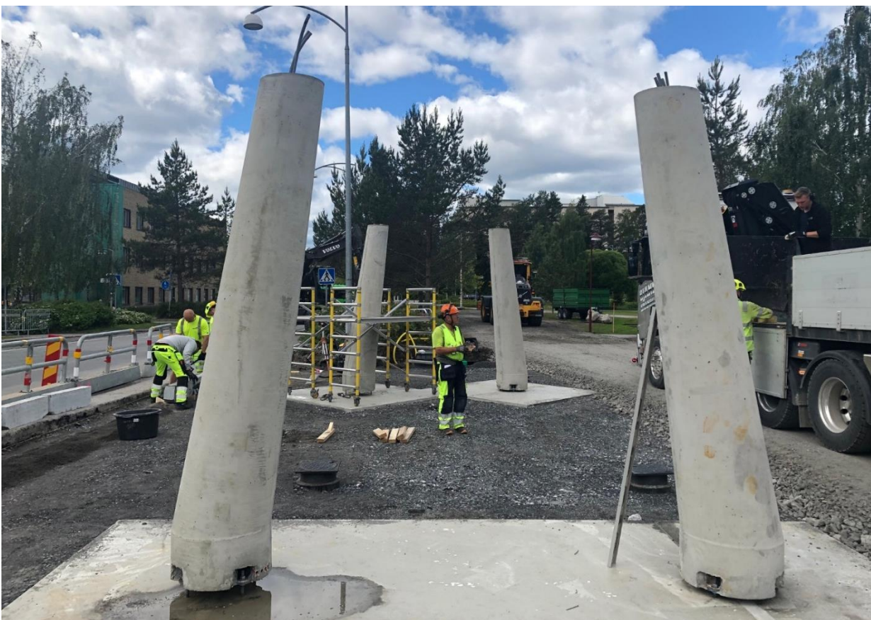
Picture 13. All pillars mounted
