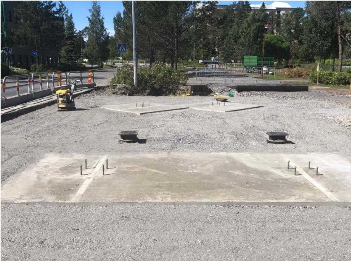
Picture 12. Mould grated and bearings packed
