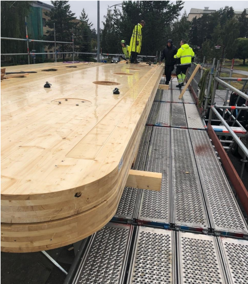
Picture 16. The top plate is mounted
