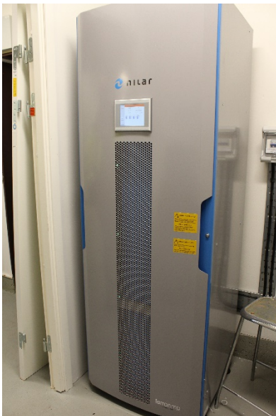
Figure 4. Installed battery storage at the campus of Umeå.
