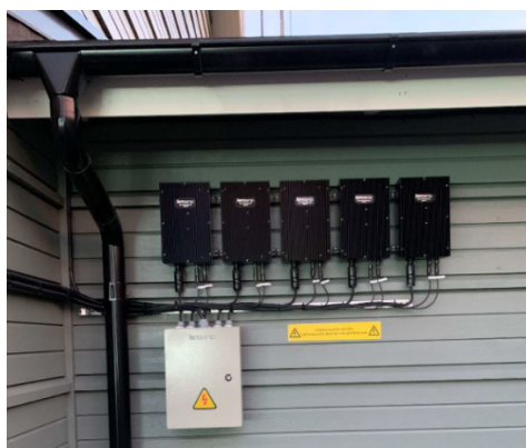
Figure 3. Installed solar optimizer at the campus of Umea.
