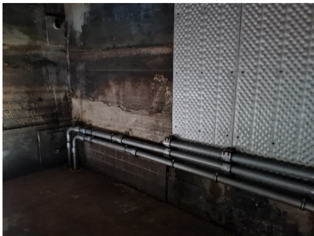
Figure 11: Panels and pipelines of the thermal energy from waste streams. Source: City of Rotterdam
