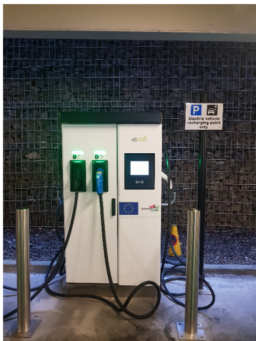
Figure 43: EV- charging point
