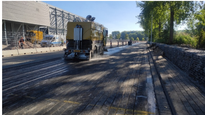
Figure 12: Asphalt milling of the pavement. Source: City of Rotterdam
