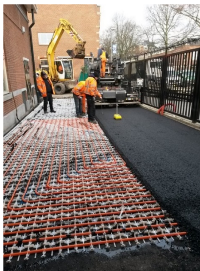
Figure 5. Asphalt collector at demonstration site, pumping station Wolphaertsbocht.
