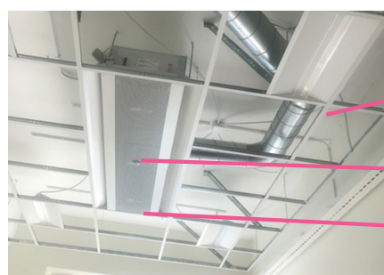
Figure 8: Smart system components: The intelligent building control includes sensors, lighting, and the chilled beam which allows control temperature and ventilation.
